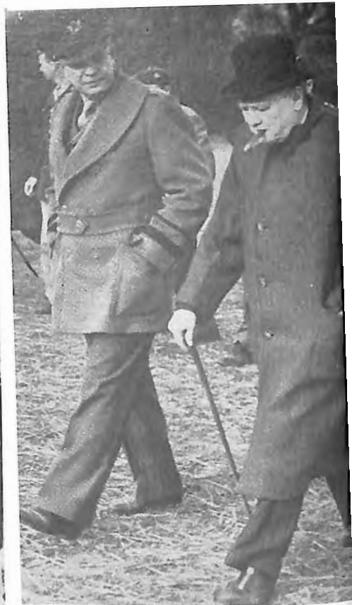
Churchill on inspection with Eisenhower
