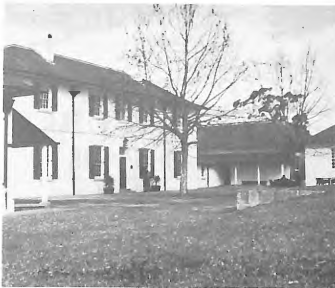
View across Courtyard showing Governor Macquarie's extension, rear of Central (main) House, kitchen wing at right with verandah and Governors suite of private rooms extreme left.
