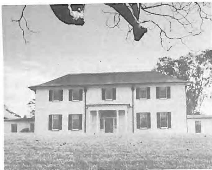
View of the front elevation showing the Central (main) portion of the House. This portion was built for Governor Hunter c. 1799. Colonnade to right leads to the Governor's Private Suite (After Governor Macquarie). The Colonnade to the left leads to the Servants Hall and Kitchen (After Governor Macquarie). Portico by Francis Greenway, convict architect.
