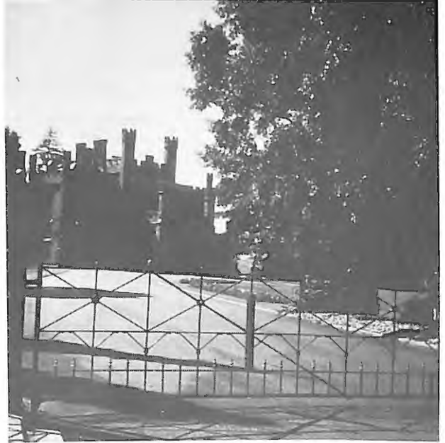
Front view from Entrance gates show the solid Gothic design of the building and Front Portico, which was added in 1873.
