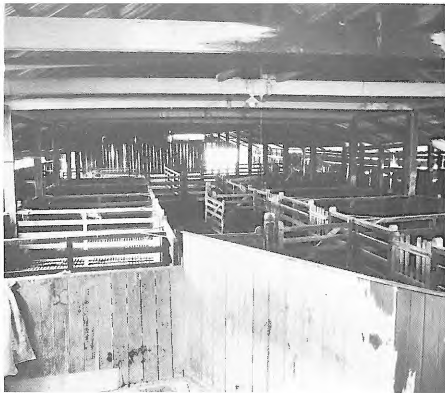
The catching and forcing pens in the eastern wing of the woolshed looking from the centre.
