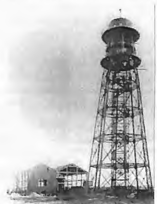
Cardington mast and winch houses under construction.
