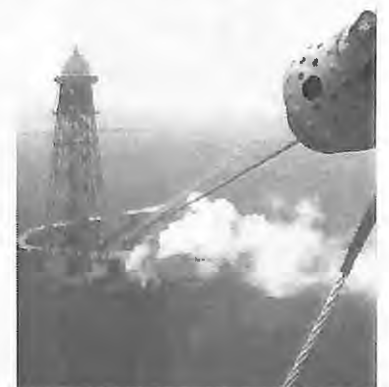
View of the mast from the nose of the R101. Steam from the winch houses can be clearly seen.
