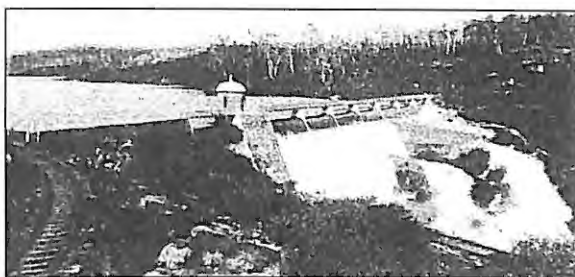
MUNDARING WEIR (HELENA DAM) OVERFLOWING Probably photographed on the first occasion, September 1903.
