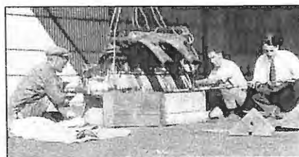
Engineers working on a Beadmore engine FK8 in Longreach hangar 1923. Arthur Baird centre back
