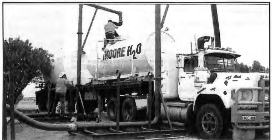
A water tanker loads up at the Merredin desalination site
