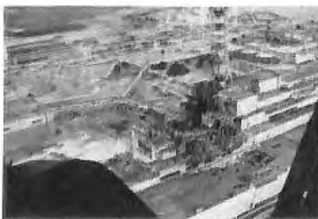
The damaged Chernobyl nuclear power plant after the 1986 explosion
