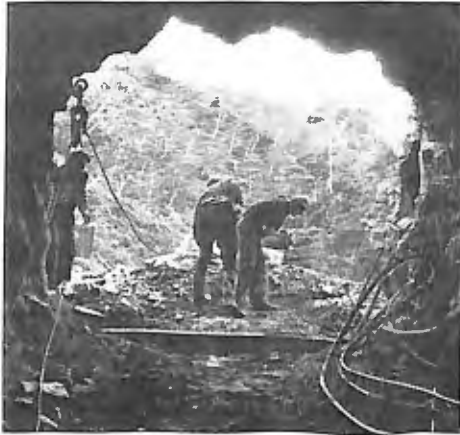
Two New Australians at work on the scheme in 1953.
