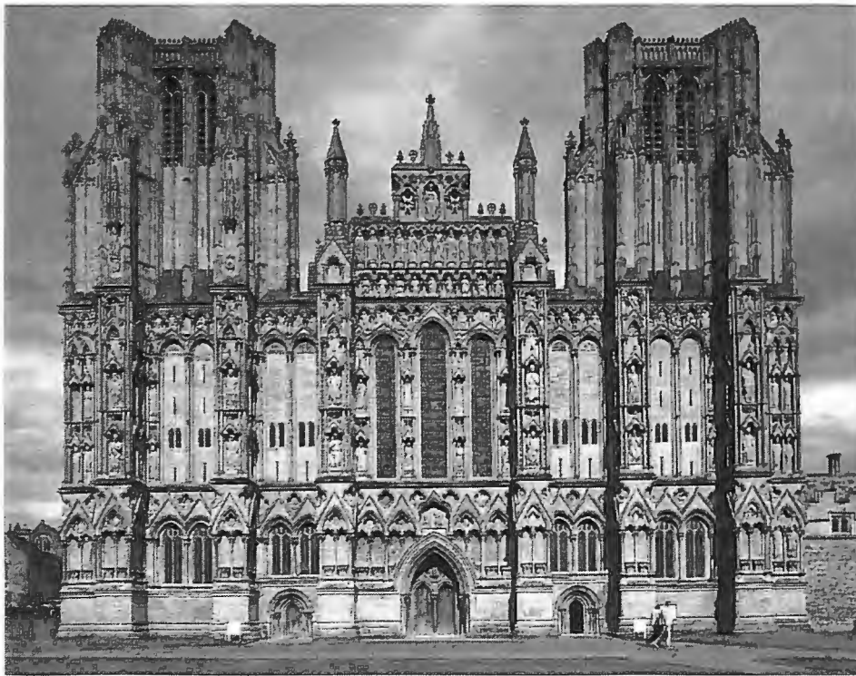
The magnificent west front of Wells Cathedral in Somerset which contains 297 superb mediaeval figure sculptures. The towers were added in the late 14th and early 15th centuries to support spires that were never built.
