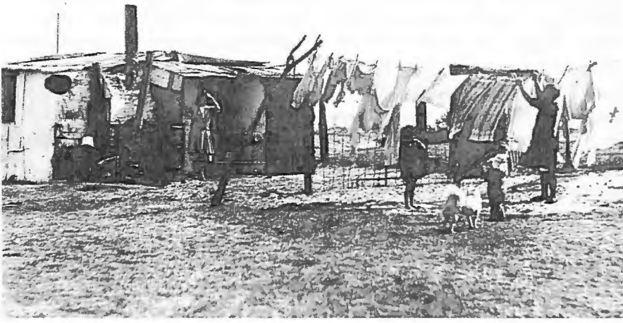
The scrubby sandhills of Sydney's seaside fringes erupted into a rash of shacks and tents that housed unemployed workers and their families who had been evicted. Shacks were built in any materials that came to hand, including old rotten timber and sacks waterproofed with lime and fat.
