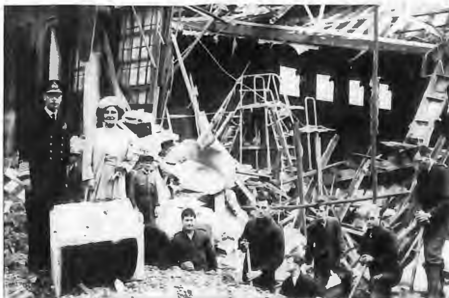
September 1940: Their Majesties view bomb damage to Buckingham Palace.
