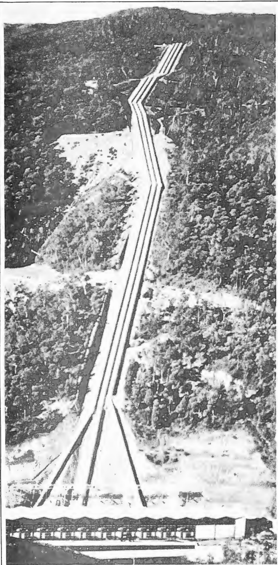
Part of the Snowy Mountain Hydro-Electric Scheme.
