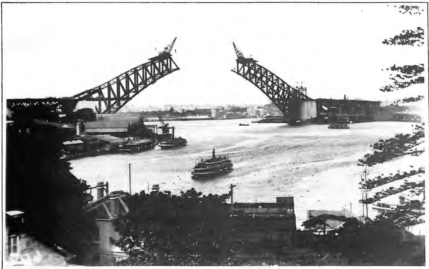
Sydney Harbour Bridge under construction. It was opened in 1932.
