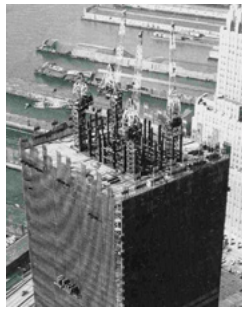
WTC 1 during construction.
