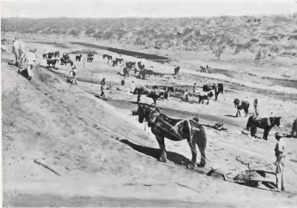
TRANS-AUSTRALIAN RAILWAY—SCOOPING TO FORM EMBANKMENT.
