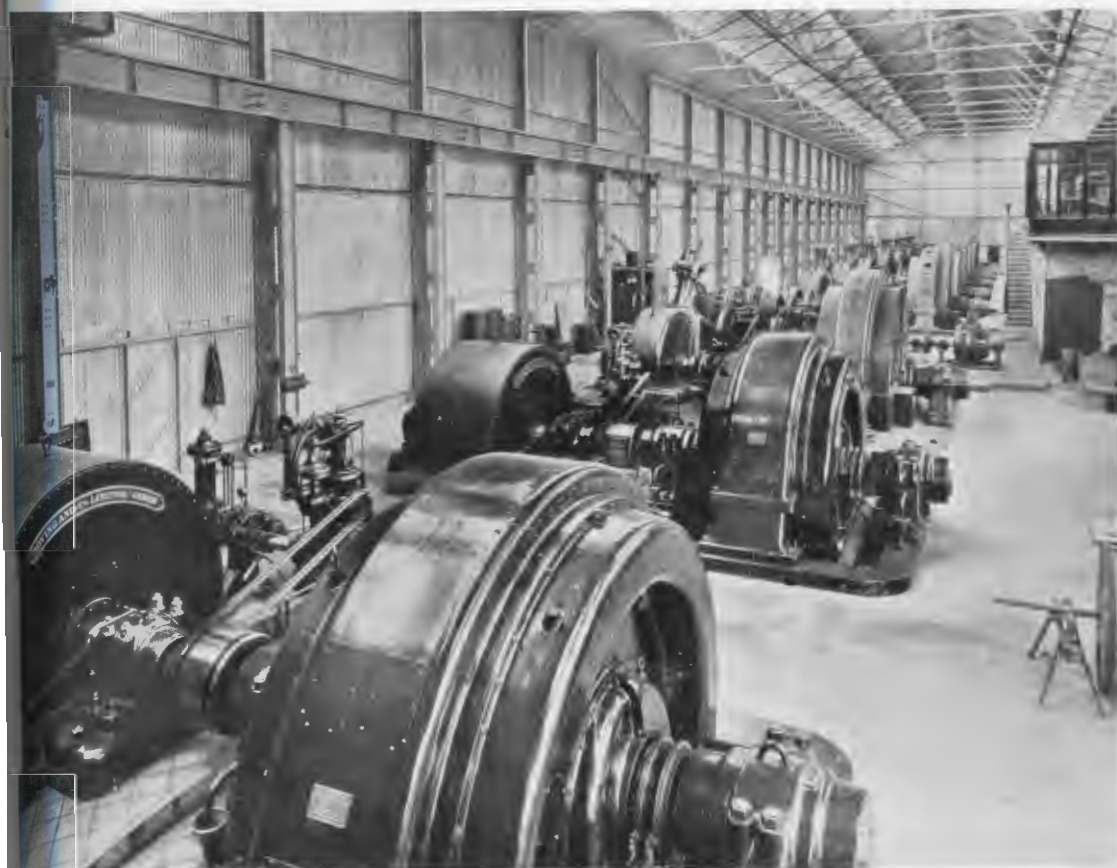
NINE TURBINES, GENERATING 66,000 HORSE POWER.
