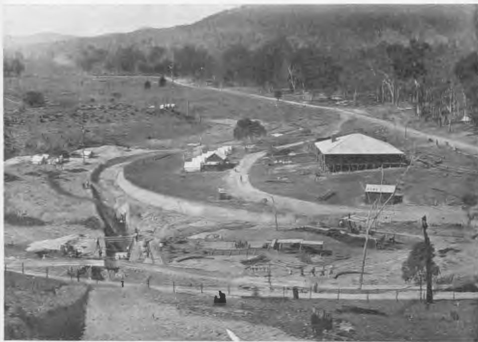
NYMBOIDA HYDRO-ELECTRIC SCHEME—CANAL IN COURSE OF CONSTRUCTION LEADING FROM RIVER.
