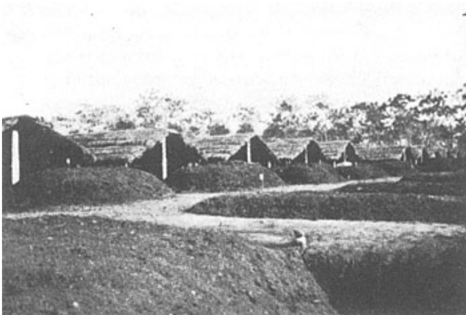
Covered and uncovered pits.
