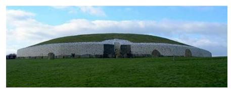
Newgrange barrow mound in County Meath, Ireland. Constructed in approximately 2500 BC, it is one of the finest passage graves in Western Europe, 250 feet (76 m) across and 40 feet (12 m) high. It was so constructed that at noon on the winter solstice, the sun shines through a specially made slot just above the entrance, directing rays into the furthest recesses of the tomb. The splendid construction is a tribute to the early white builders of Neolithic Ireland.
