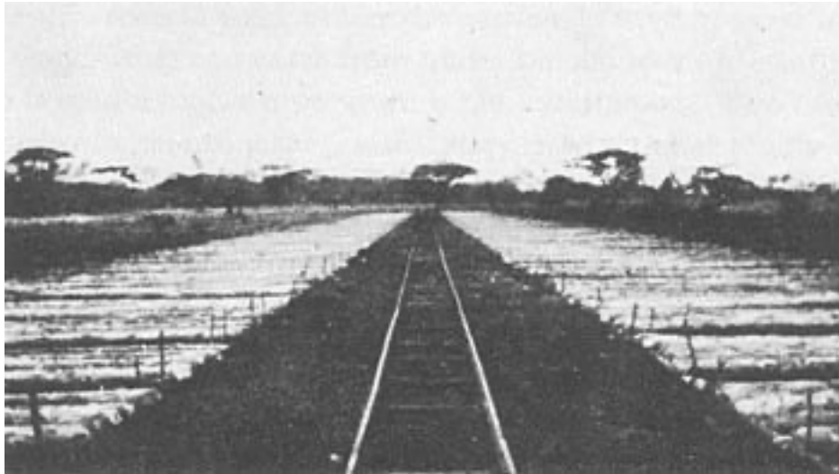
Light railway and foundation of sisal poles.
