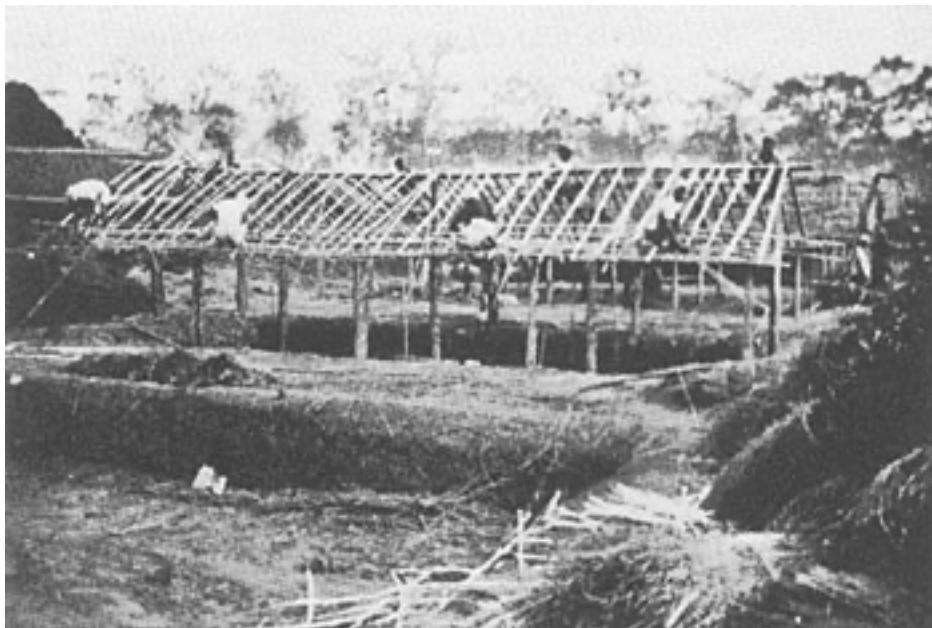
Roofing a pit.
