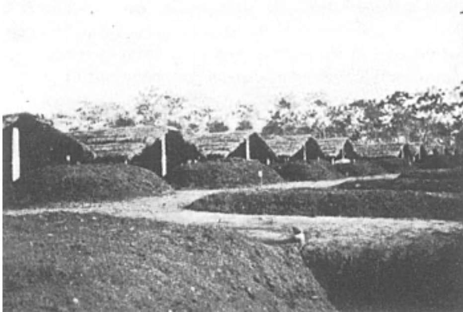
Covered and uncovered pits.
