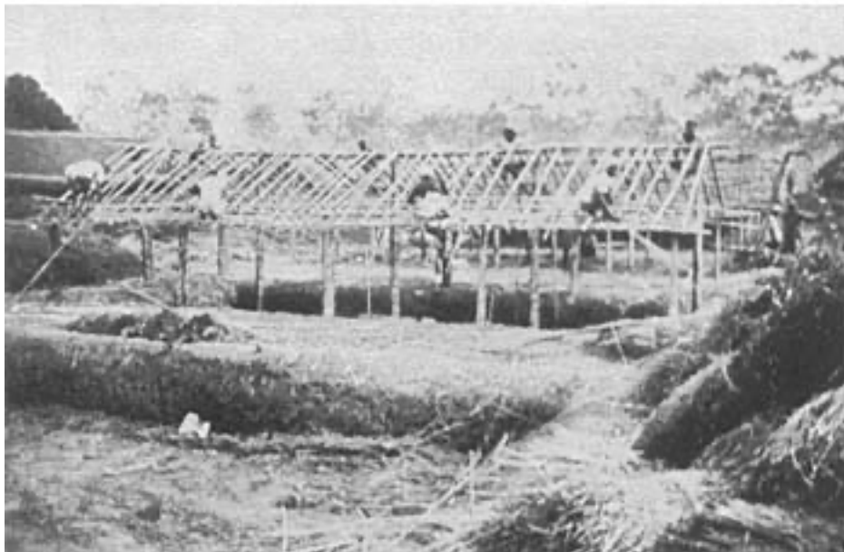
Plate VIII. Composting at Gandrapara. Above -- Covered and uncovered pits; Below -- Roofing a pit.
