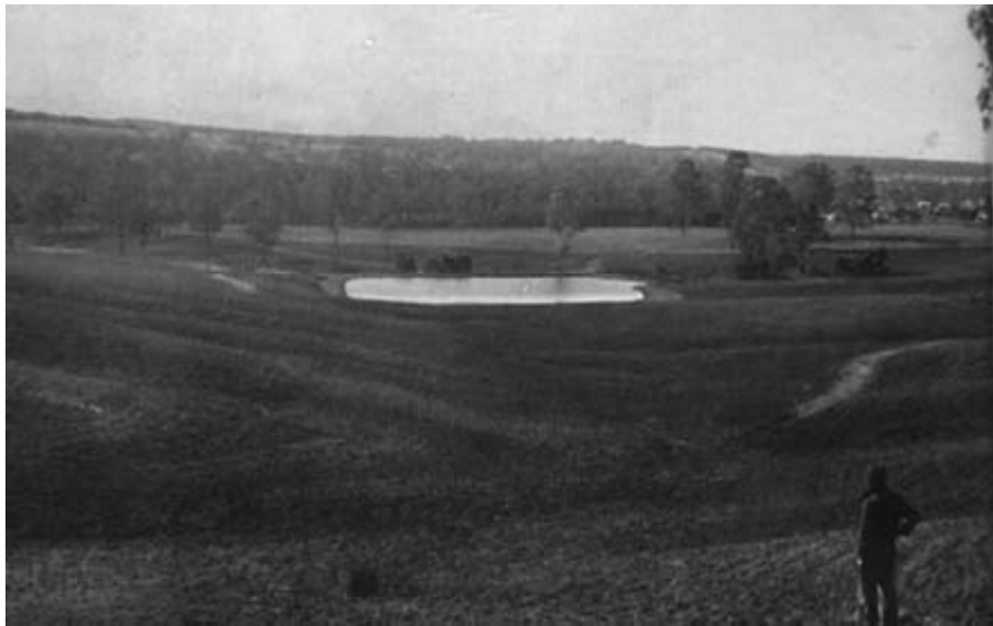
Plate 5: "Conversion-year" cultivation and erosion holes plowed out by the "Graham". "Pelican Rest" dam, built before Keyline was originated, has a 4-inch outlet.
