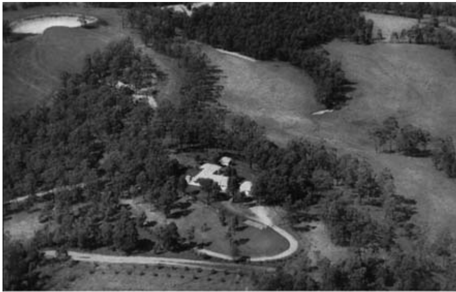
Plate 2: Aerial view of "Nevallan" homestead, with High Contour dam in the top left-hand corner of the picture. This dam, which is filled by drains, collectes its water from the roads and yards of the homestead area. It has 4-inch outlets through the end walls.
