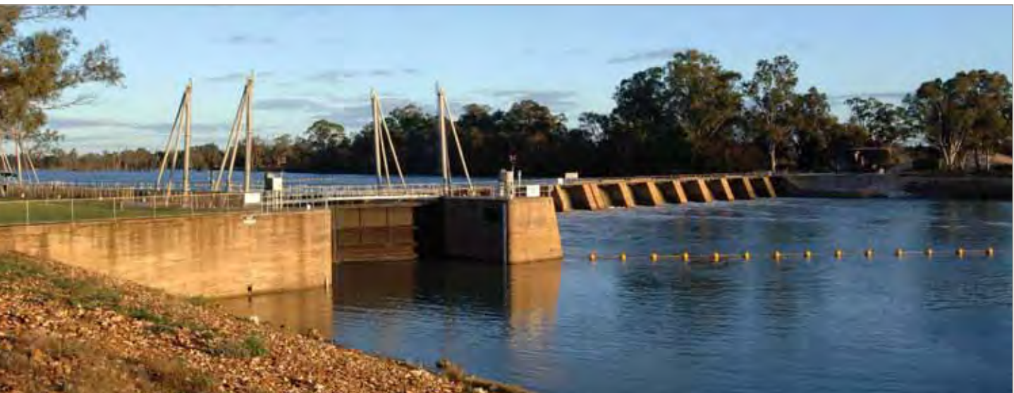
Lock 4 on the River Murray at Berri, South Australia
