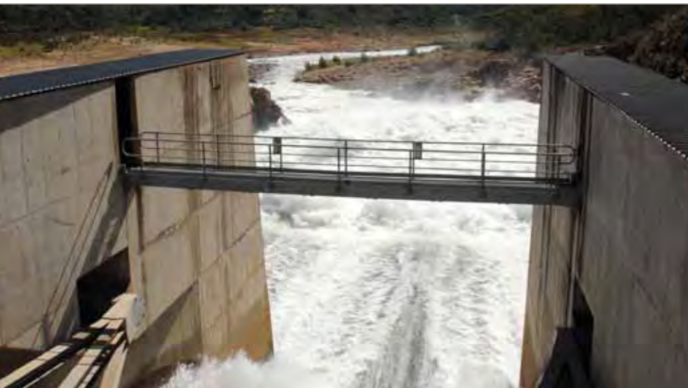
Release of water from Jounama Dam into Blowering Dam, New South Wales
