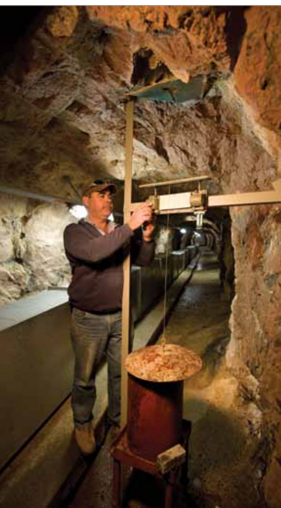
Measuring water seepage at Burrinjuck Dam, New South Wales
