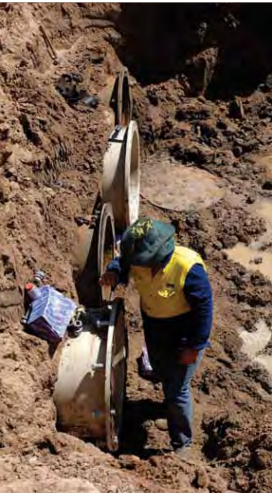
Diversion channel used to take water to Buckinbah Weir, Queensland
