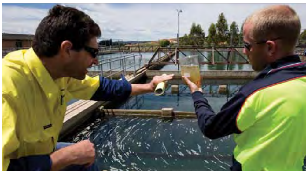
Taking measurements at the sedimentation and flocculation tanks, Bathurst Water Treatment Plant, New South Wales
