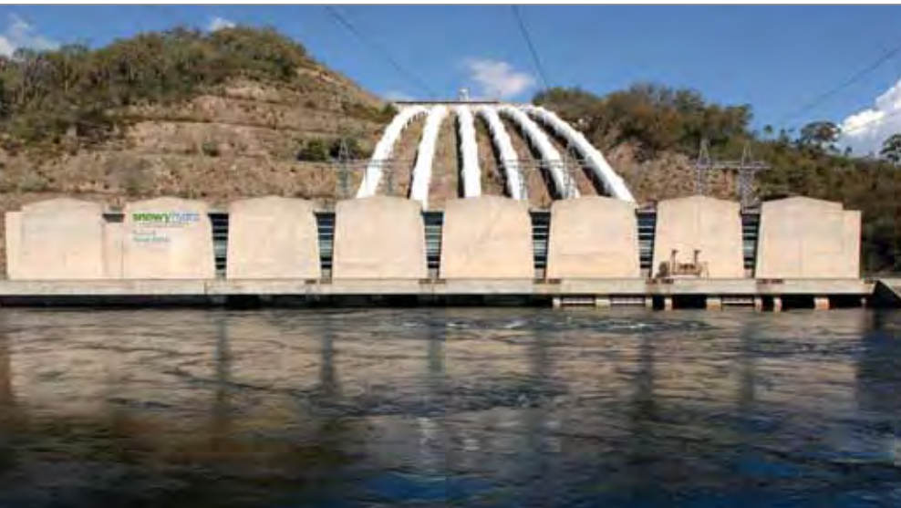
Tumut 3 power station, part of the Snowy Mountains Scheme near Talbingo, New South Wales
