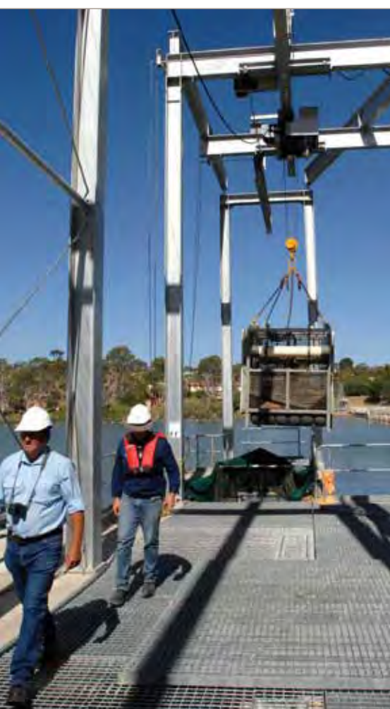
Fishway and carp separation trap on the River Murray at Lock 1, Blanchetown, South Australia. Native fish can swim through, while carp are caught and processed for bait to be used in the fishing industry
