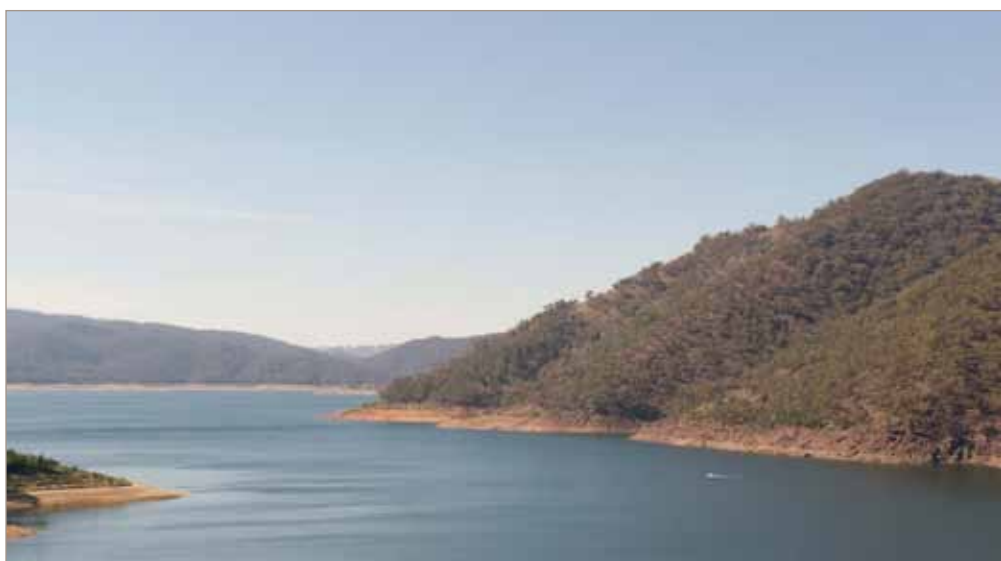
Burrinjuck Dam in New South Wales at 38.6% capacity, May 2009
