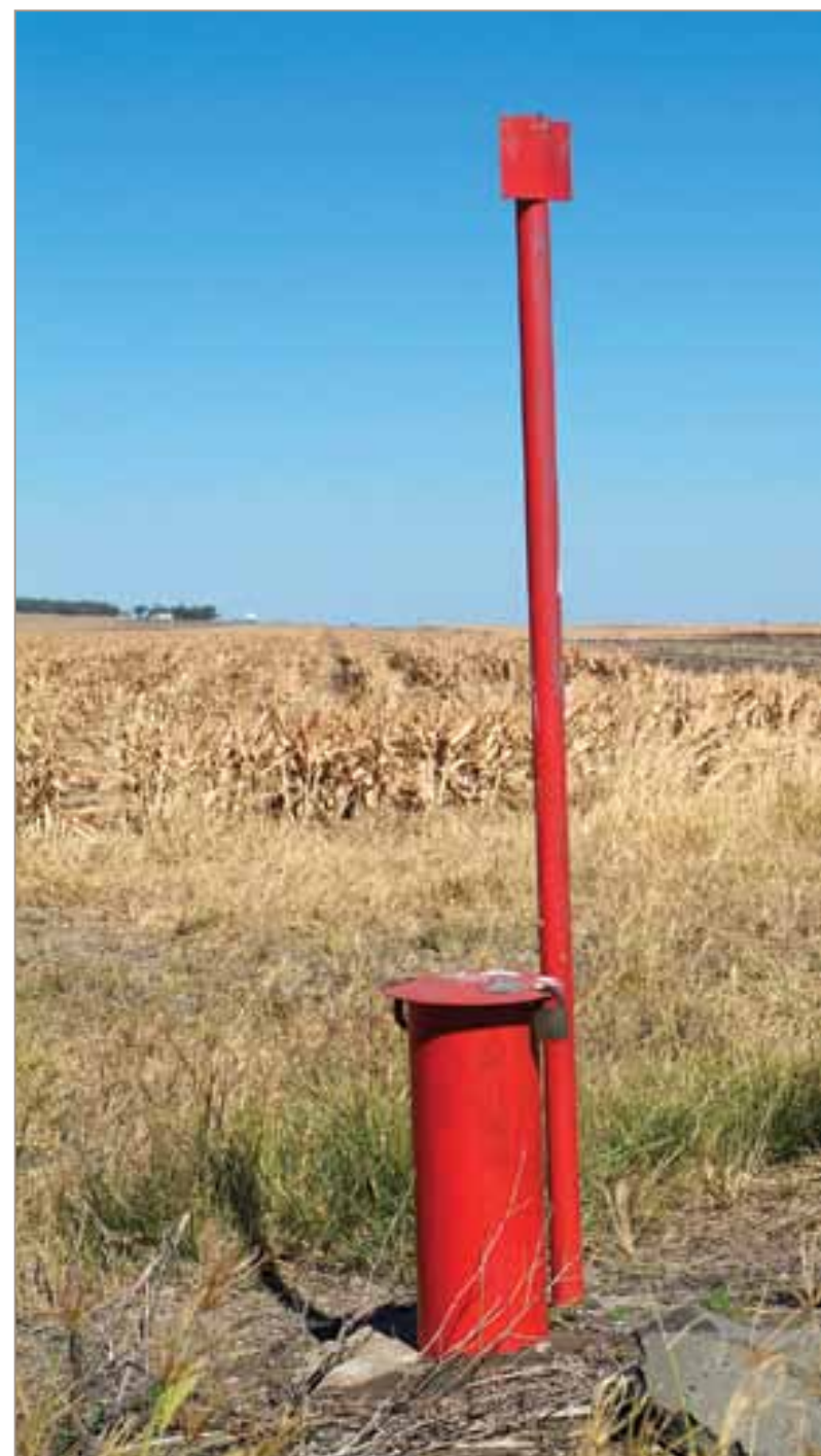
Groundwater monitoring bore on the Toowoomba–Cecil Plains Road, Queensland
