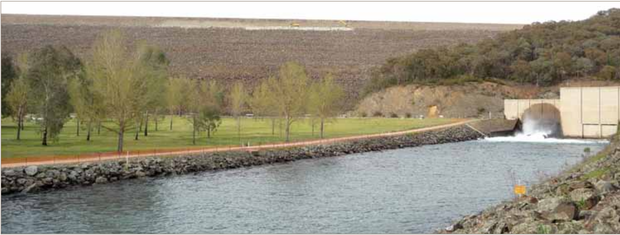
Blowering Dam near Tumut, New South Wales
