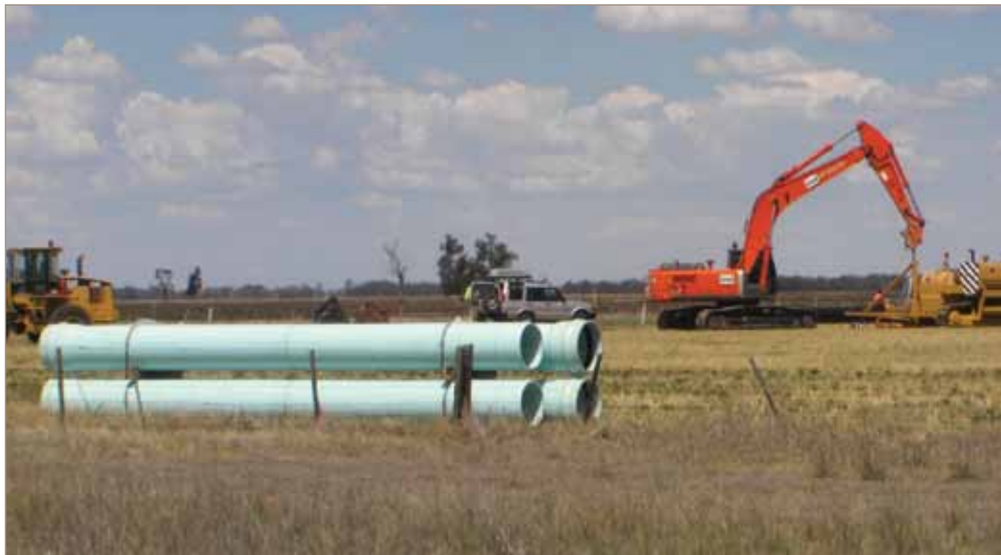
Wimmera Mallee Pipeline construction, Victoria
