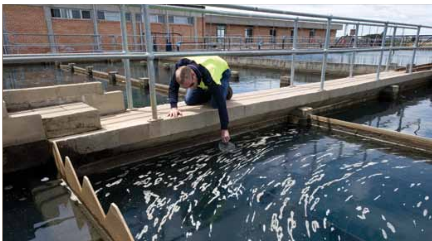
Testing the water of sedimentation and floccation tanks at a water treatment plant at Bathurst, New South Wales
