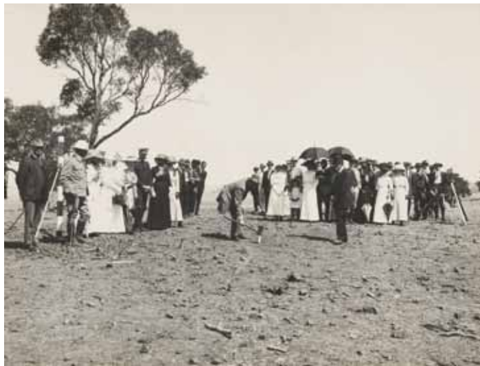
The Honourable King O'Malley, Minister of State for Home Affairs, driving the first survey peg at Canberra Hill, in connection with the lay-out of the Federal City, on 20th February, 1913, National Library of Australia.
