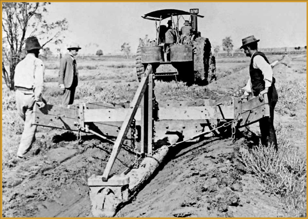
Channel construction using steam traction engine and delver ditcher, c.1918.
