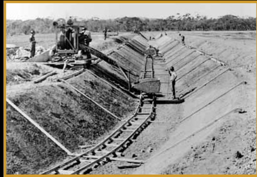
Main Canal concrete lining, looking upstream towards Three Ways Bridge c.1923
