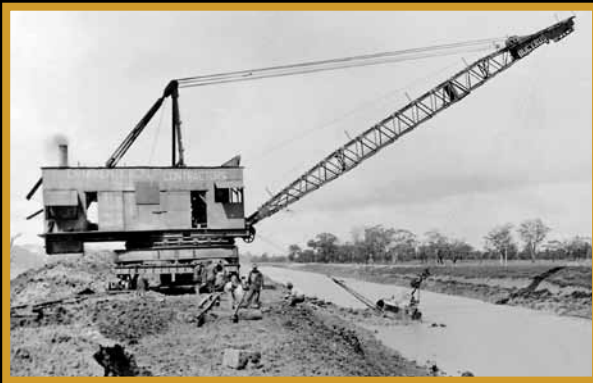
Widening of Main Canal, c.1920. The Main Canal was widened to ensure there was enough water for soldier settlers' farms.
