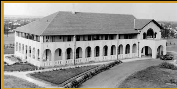
Hydro Accommodation House, Leeton, for WC&IC officers and visitors, c.1920.
