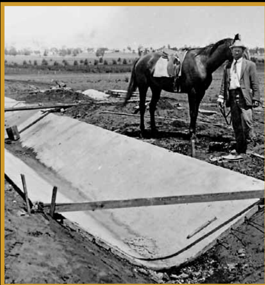
Constructing concrete lined distribution channel c.1912
