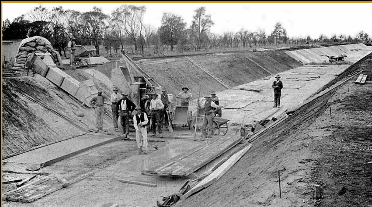
Main Canal concrete lining c.1916. (J Degotardi, John Newland collection)
