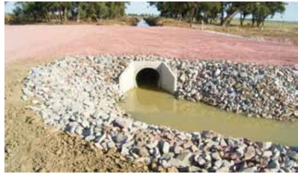
Yanco Main southern drain culvert.
