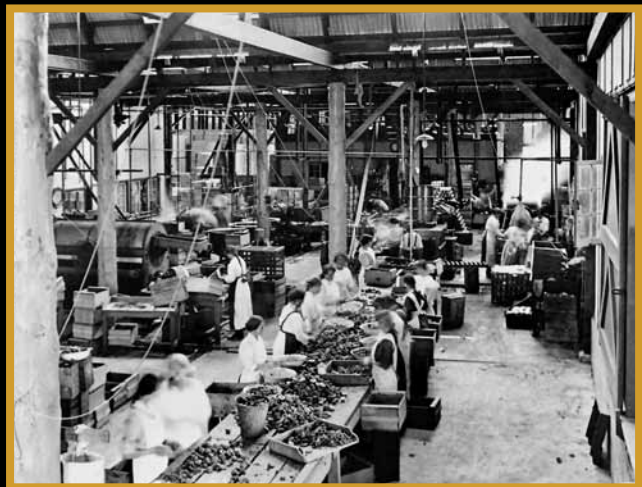
Interior of WC&IC Canning Factory at Leeton, preparing fruit for canning, c.1915.
