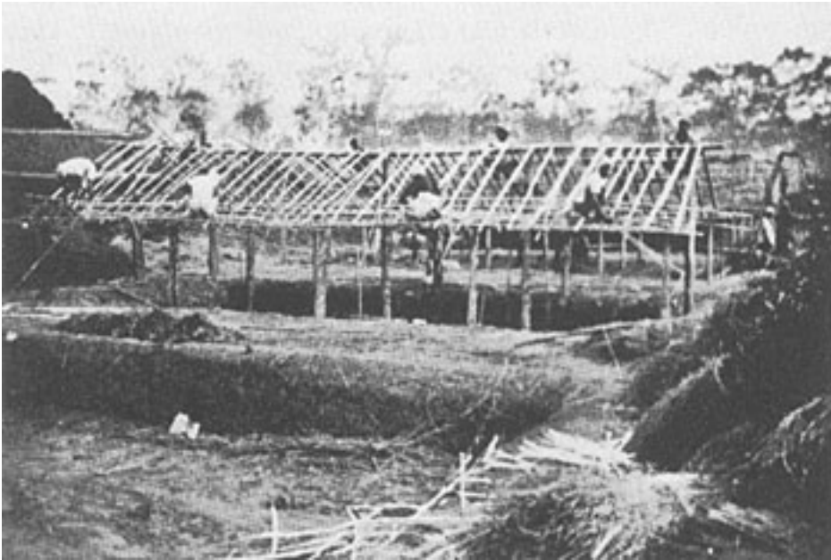
Roofing a pit.
